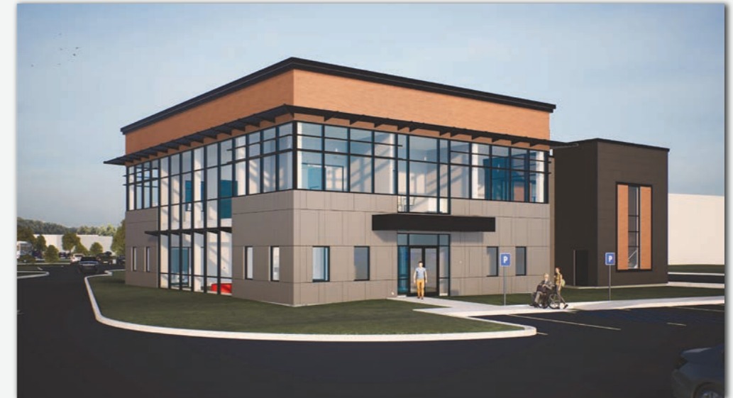
Our new headquarters is currently under construction, with opening planned for 2027.
